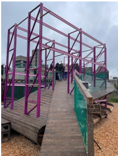
Figure 19: Leuven – Reclaimed materials used for the construction of the Olevodroom
