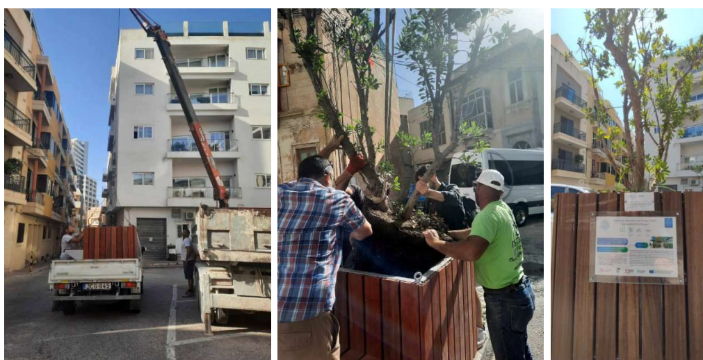
Figure 30: Gzira (MT)- Execution phase - Planters and trees being delivered to the site and installed
